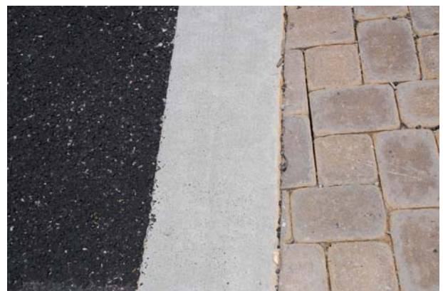
Figure 3: Porous Asphalt and pervious pavers
