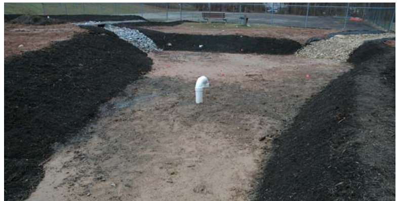
Figure 1: (top) Bio-retention area in the rain Figure 2: (bottom) Bio-retention under construction, white pipe is the overflow device, engineered soil mix has been placed over the underdrain system
